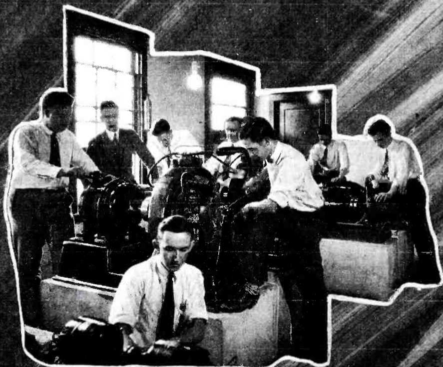
BROADCAST STATION KMOX - ST. LOUIS, MO. OPERATING STAFF AT WORK ON GENERATORS
